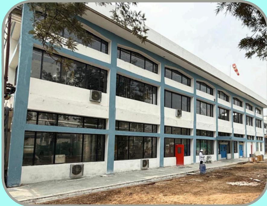
P-8 Plant Expansion Completed
