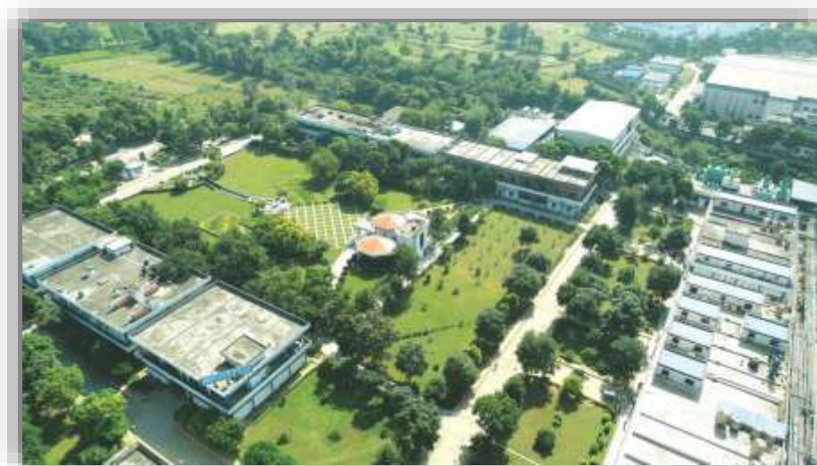
Baddi API Plant: Arial View
